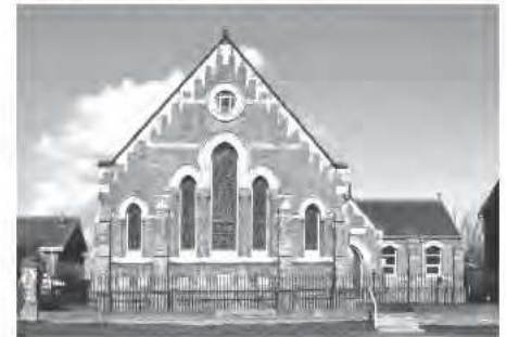
The new chapel as used from 1895- 2011 Photo © Brian Mossemenear
